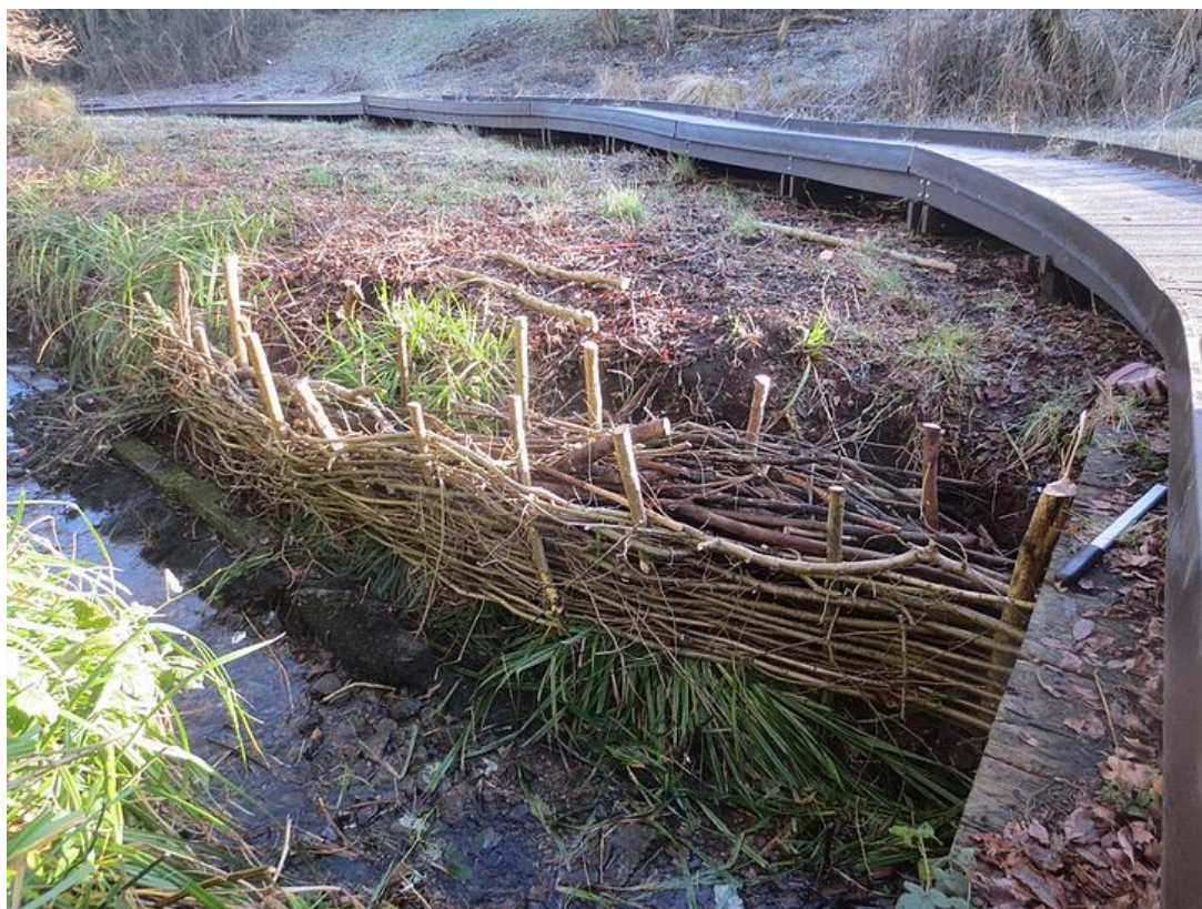
Hazel wattle structure and cut material used in bank restoration
